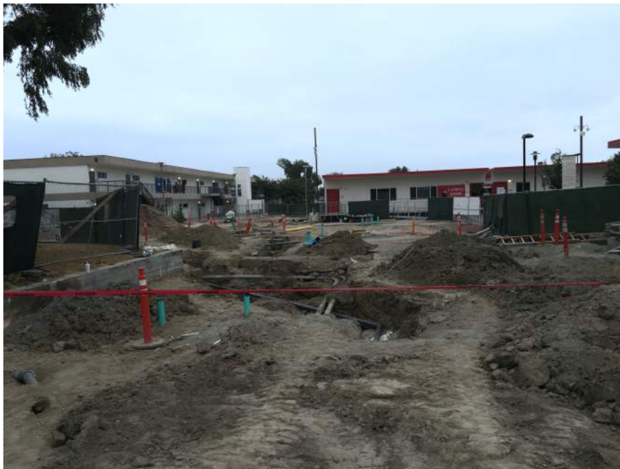
Phase 4 Construction Zone
