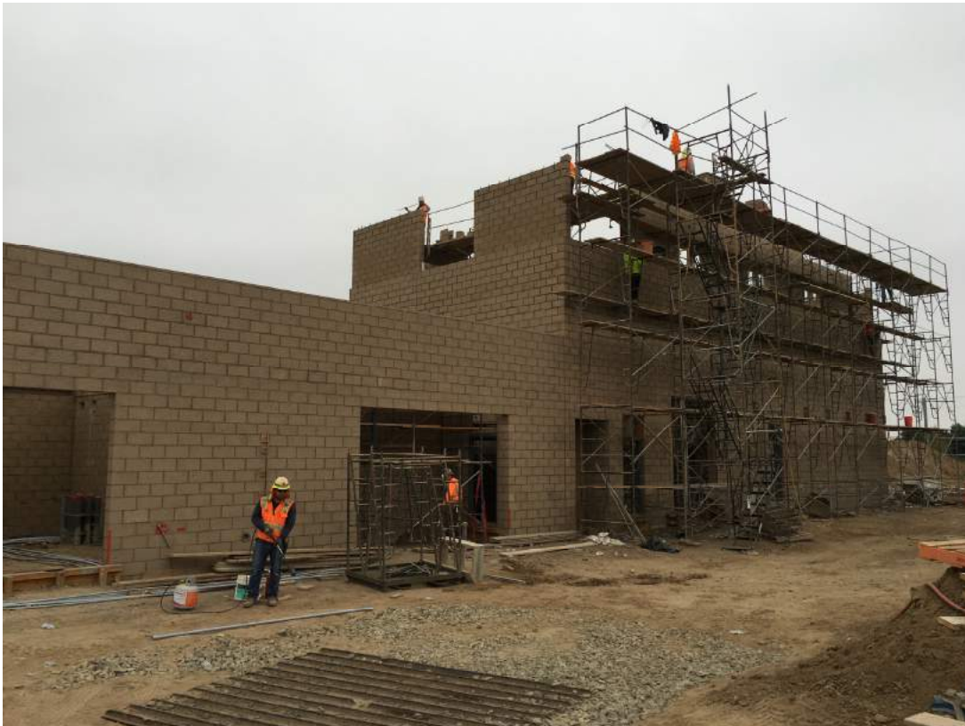
Central Plant Construction Zone
